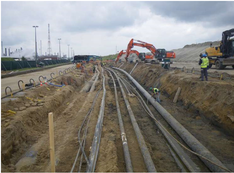
Figure 2.5 Repair works to secure the pipelines and restore the bed.
