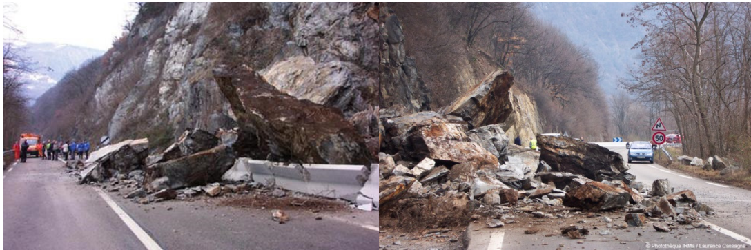
Figure 2.15 On 24/01/2004 a 200-ton rock fall occurred on road RN91 (now called RD 1091), which blocked this national road for more than 24 hours and imposed traffic deviation, while many people were travelling to ski stations (pictures from L. Cassagne, Irma 21 ).
