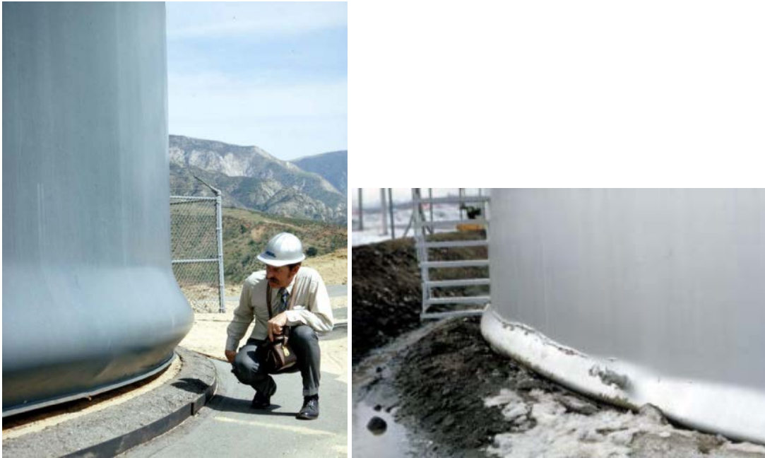
Figure A2-42 Buckling of the shell at the base of a tank after an earthquake.
