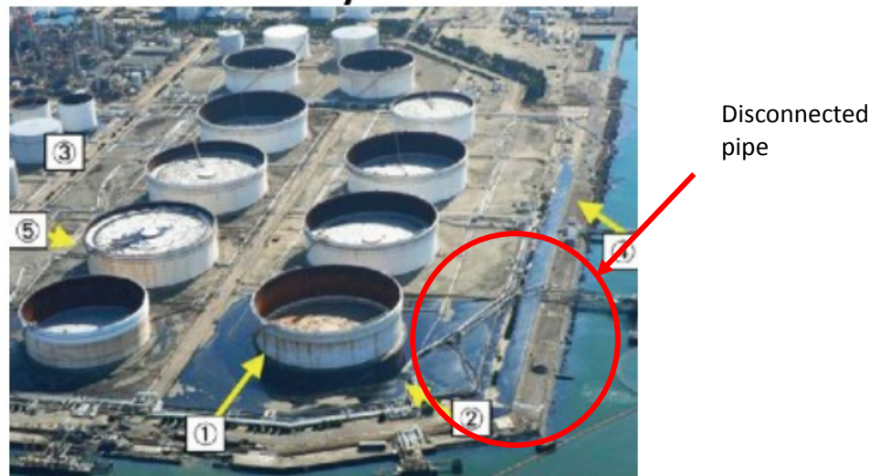
Figure A2-40 Deformation of a pipe impacted by the walls of a retention pond after they were torn out of the ground.
